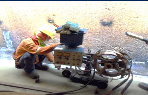
SAW(LT-7) Bottom and Corner Joint Welding
