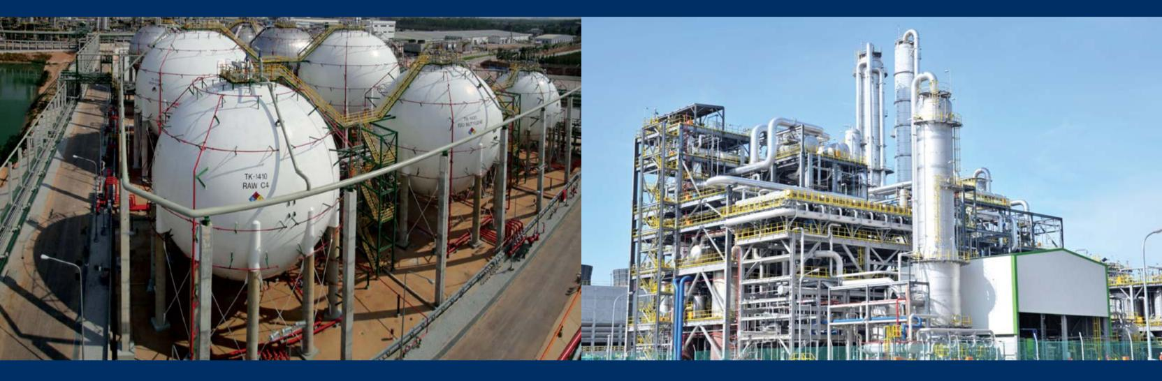
Map Ta Phut Olefins Chemical Complex tank farm unit is used for the storage and distribution of various chemical products such as naphtha, HP ethylene, HP propylene, raw/mixed C4, cracker bottom, gasoline and aromatics.
