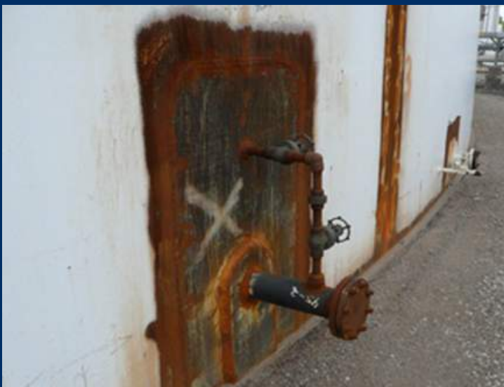
Repair and replacement of tank shell/roof nozzles, manways, venting system (gauge hatch, PV, PVRV, ERV, etc.).
