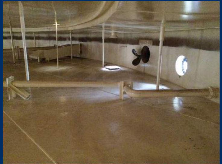
Repair and replacement of internal tank pipe heating coil, sparger pipe system, water draw-off piping.
