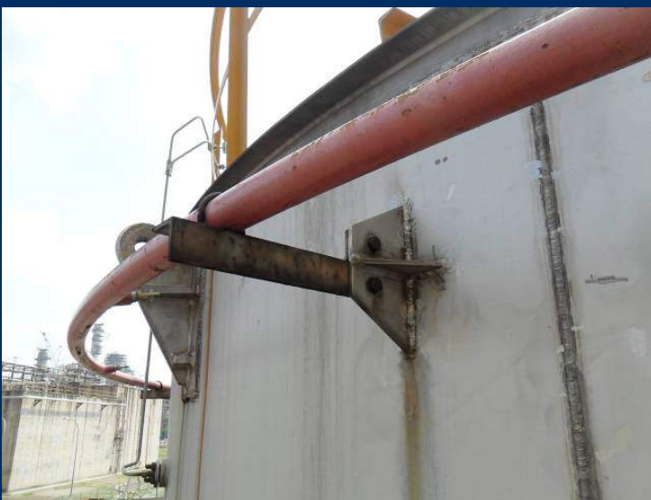
Repair and replacement of fire water/foam pipe system.
