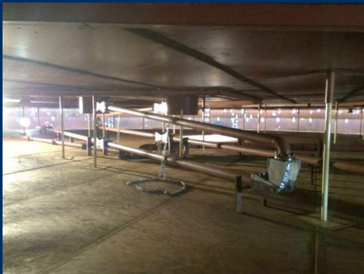
Repair and replacement of floating roof drain system, rolling ladder.
